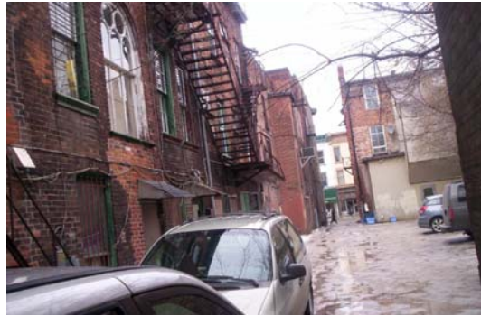
Rear alley looking towards Hunter Street.
